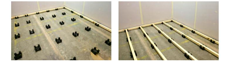
The Cradle system is designed to take a **uniformly distributed load of 5kN = 509kg**. This load can be increased because of the system flexibility.
